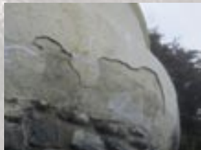
Railing and stucco repairs from April, 2010
